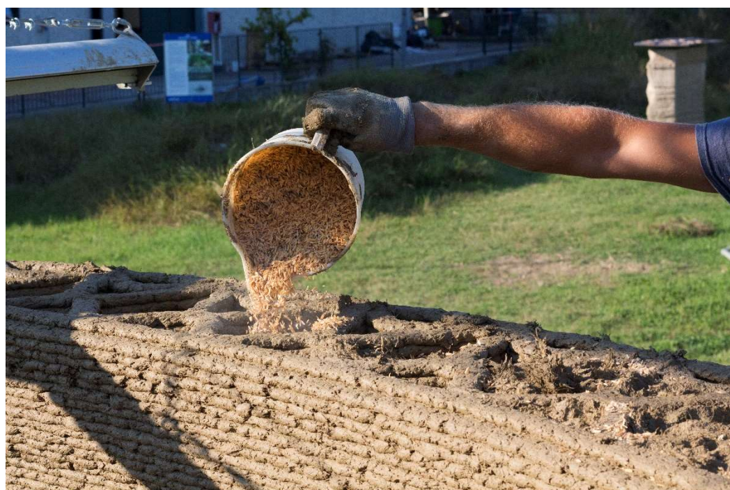
Figure S4. Filling of Gaia's honeycomb structure with rice husk [source WASP].
