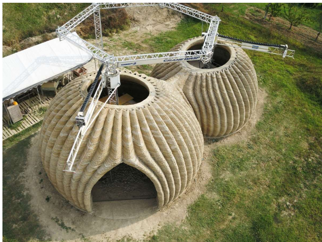
Figure S8. The two domes of Tecla in an advanced stage of completion [source WASP].
