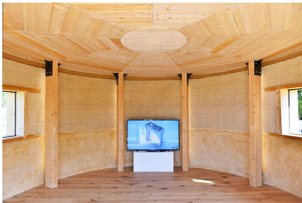
Figure S6. Four of the eight wooden pillars that sustain Gaia's roof [source WASP].
