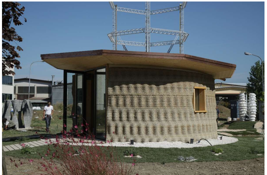
Figure S3. The Gaia House by WASP: a 3D-printed prototype constructed of biodegradable materials [source WASP].
